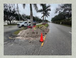
main entrance North to Bonita Beach Road are irrigated and maintained by Worthington. This irrigation piping is original and has started to have more frequent failures due to its age. Because of the road and other utilities, the pipes are
