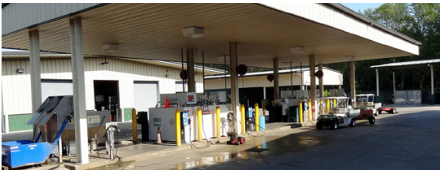
This covered equipment wash and refueling area is for a larger 36-hole facility that features a wash-water recycling system.
