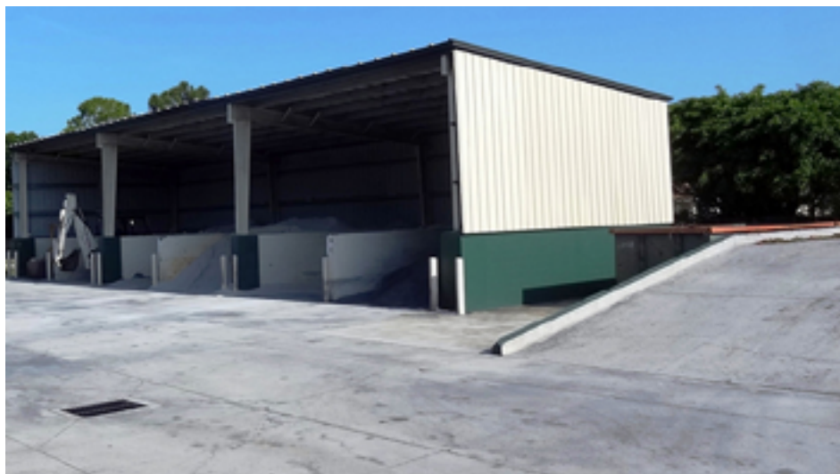
Covered bins are recommended for dry storage of bulk materials such as sand, soil, gravel, mulch, etc. They can be used to house tractors and other loading equipment as well. Notice to the right an elevated access area to allow workers to dump trash into waste receptacles.
