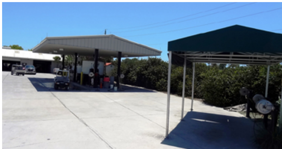
Covered equipment wash/fuel areas improve staff morale, reduce fuel evaporation, and lengthen the useful life of tanks and hoses. These areas are staged so that equipment may first be blown off with compressed air (foreground) before washing/fueling. Equipment can then be inspected by equipment managers (background) or stored.
